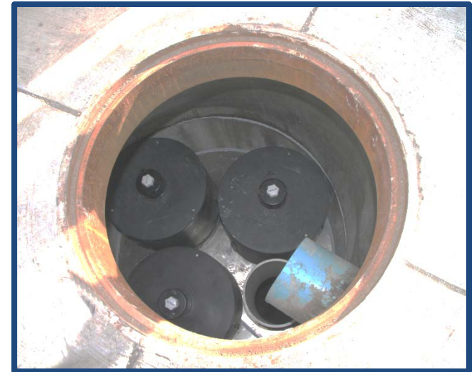
Manhole StormFilter
