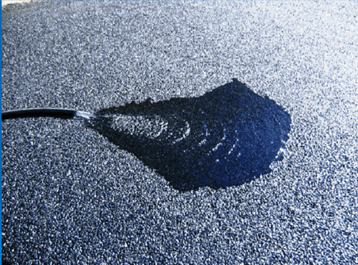
Figure 2. Infiltration of 30 gallons per minute from a 2-inch hose at UNH.
