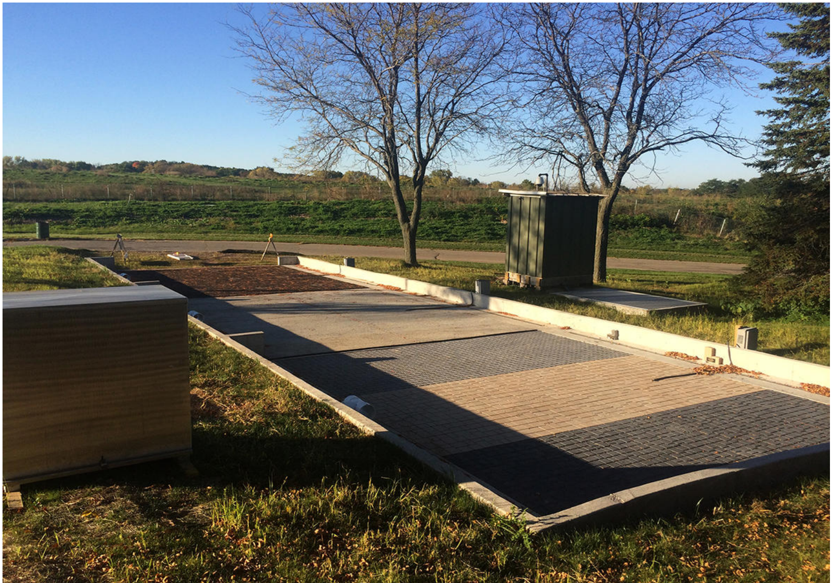
Permeable Pavement Test Site- Sycamore Avenue Madison
