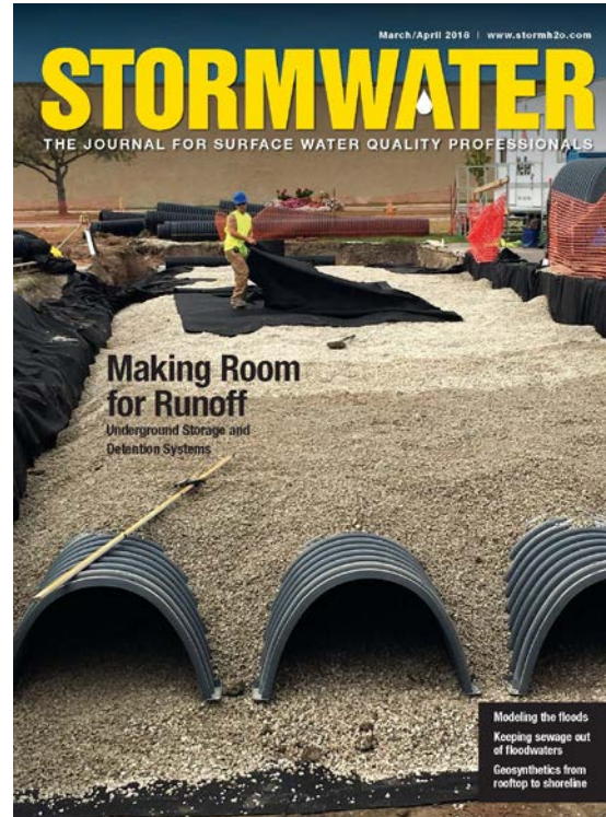
HydroStor chambers installed beneath a parking lot
