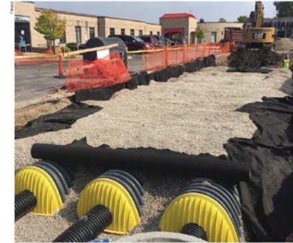
HydroStor chambers installed beneath a parking lot
