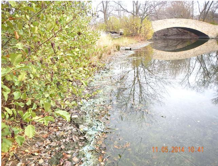
Tenney Lagoon Shoreline Stabilization
