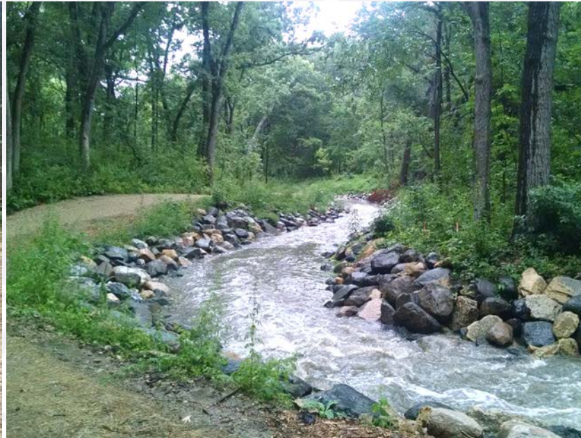
Owen Conservation Park Channel Stabilization
