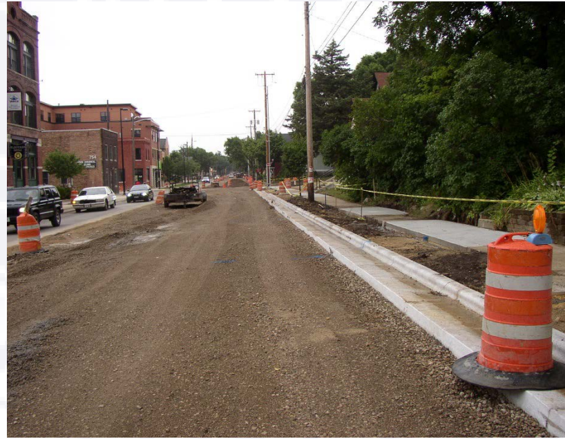
Williamson St Reconstruction
