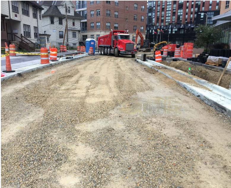
Basset St Bike Path + Reconstruction
