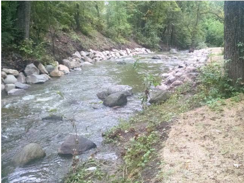
Owen Conservation Park Channel Stabilization
