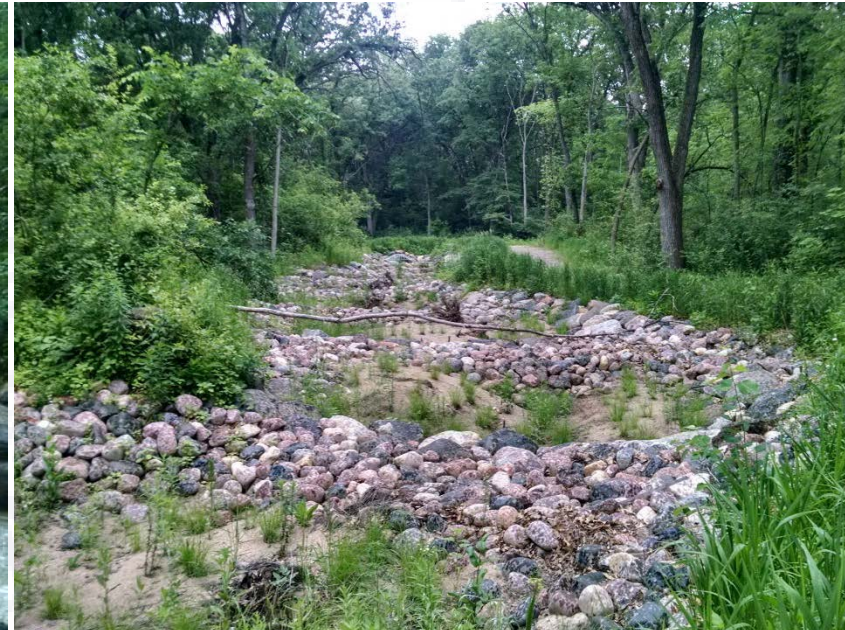
Owen Conservation Park Channel Stabilization
