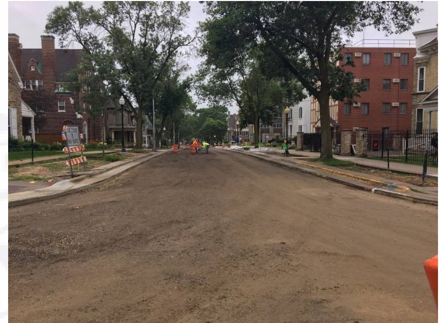
Langdon St Reconstruction
