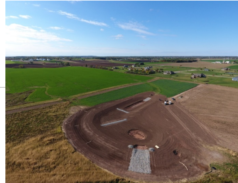
Sediment Basin - NRCS Tech Standard 350 (under construction)
