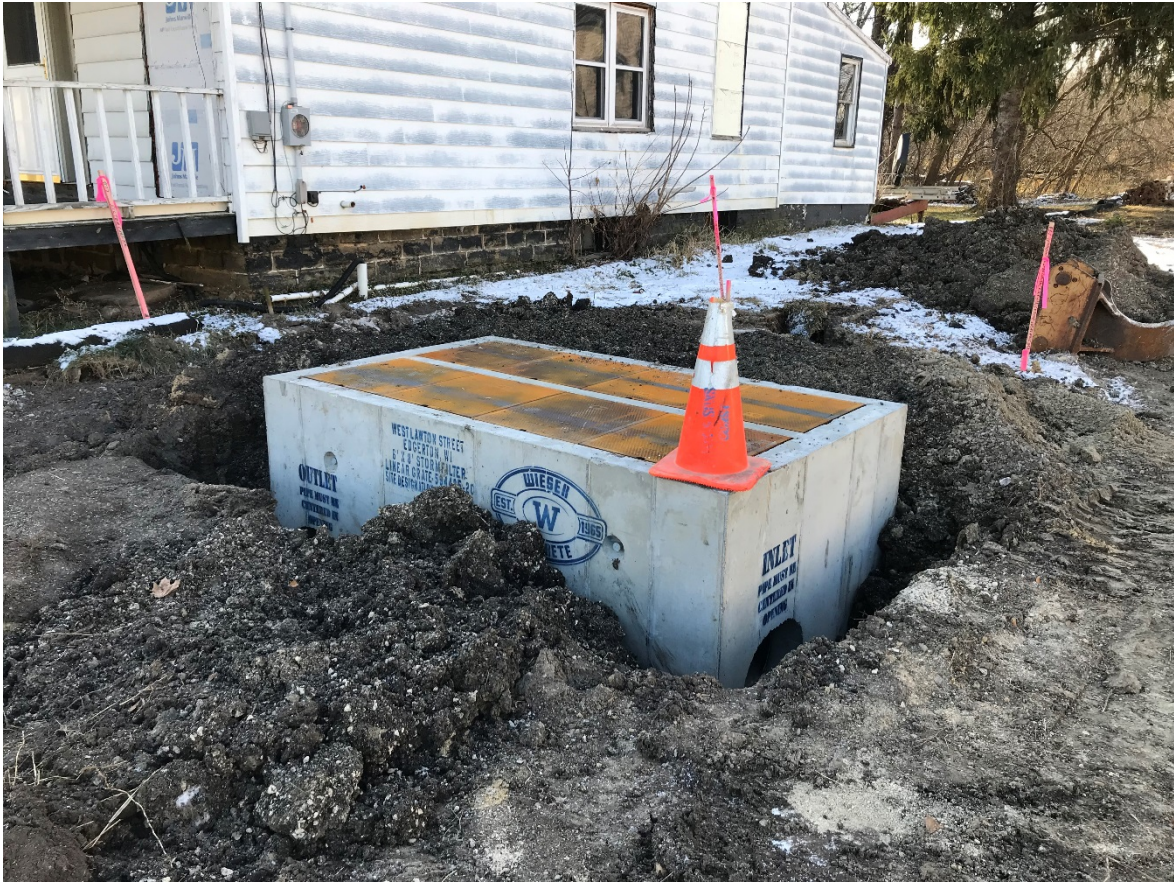
Very shallow site required used of Linear Grate StormFilter
