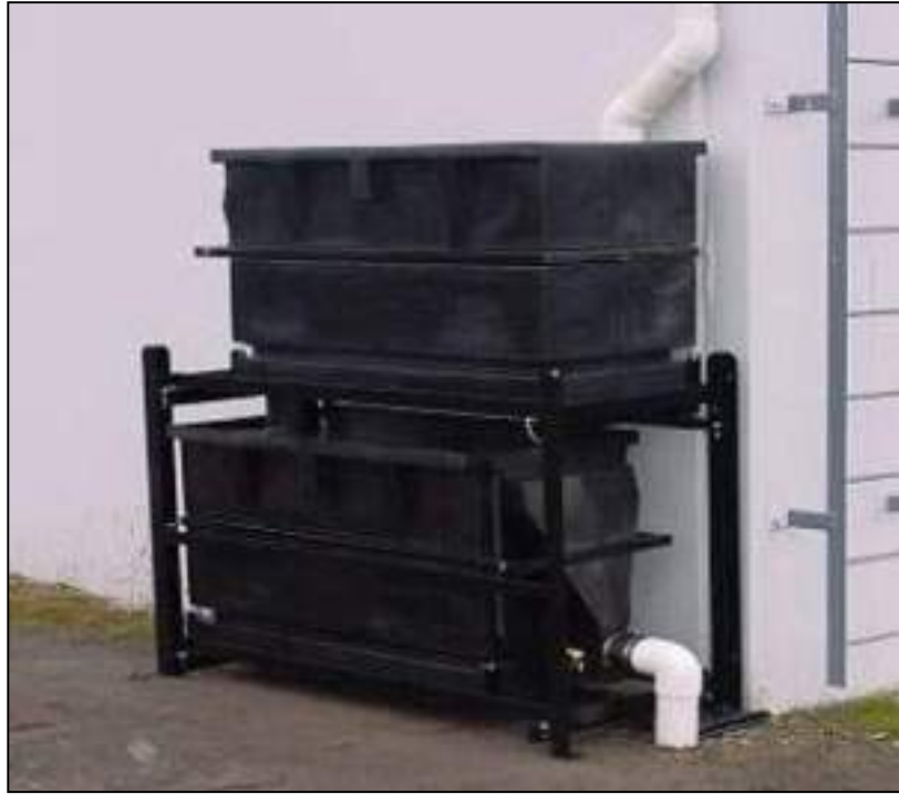
Dual-stage Up to 0.07 cfs at 15 gpm per cartridge (2 l/s at 0.95 L/s per cartridge)
