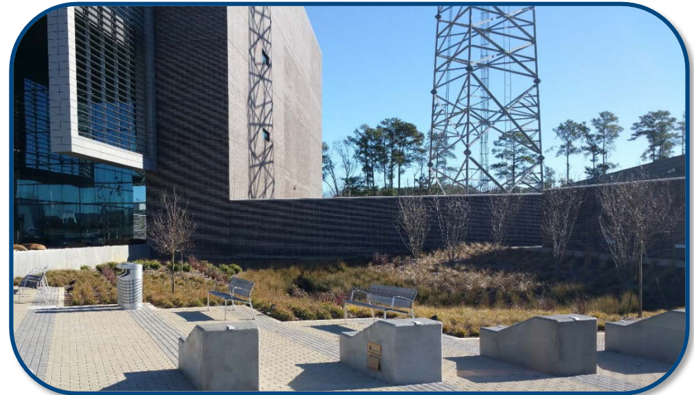
Filterra Bioscape (Emergency Communications Center– Raleigh, NC)
